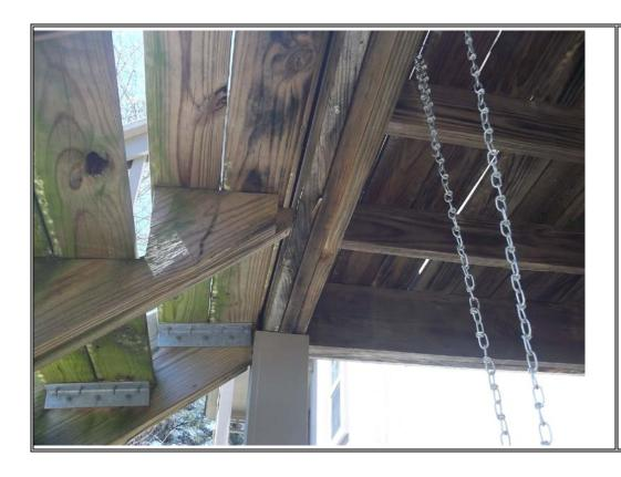
**Description:** Close up view of framing at front porch steps, center stringer not adequately attached at unit 2510-204.
