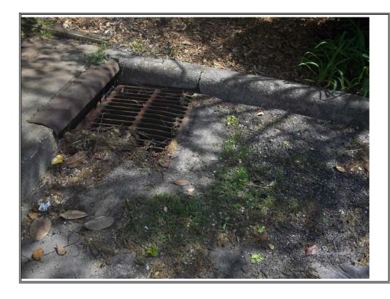
**Description:** View of sediment accumulation around inlet basin in curbing.
