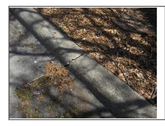
**Description:** View of cracking developing in curbing.
