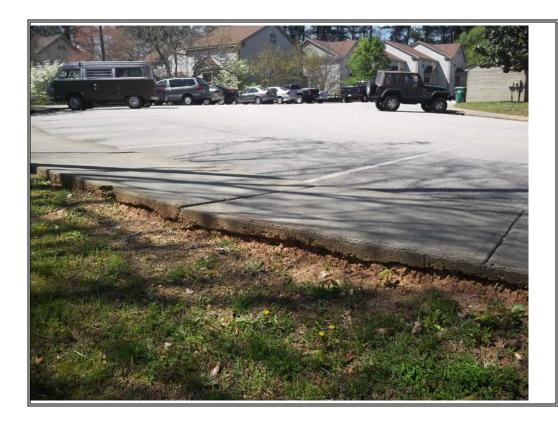
**Description:** Soil erosion undermining concrete sidewalk.
