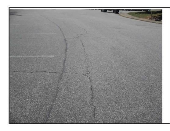
Description: View of longitudinal cracking developing in asphalt paving.
